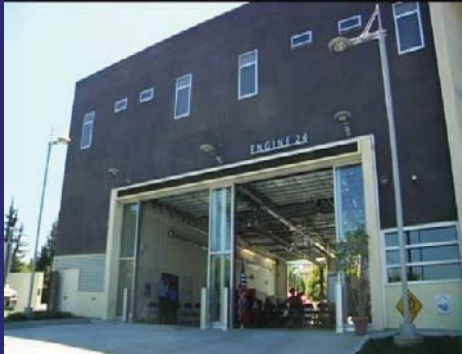
Fire Station 24 - Relocated
