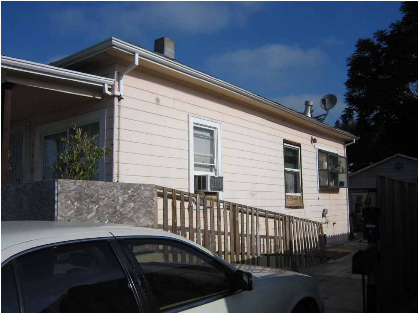
Photograph 2 815 W. San Carlos Street, San Jose View: East façade showing the ramp construction and replacement windows as well as the body of the building. Date: June 15, 2015
