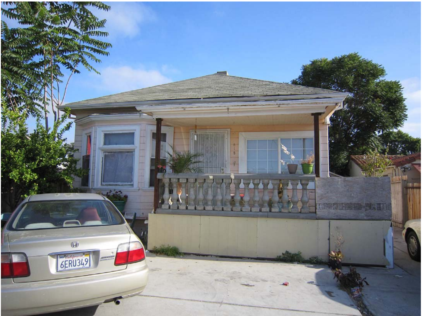
Photograph 1 815 W. San Carlos Street, San Jose View: Front façade showing the recent porch construction and replacement windows as well as the body of the building. Date: June 15, 2015
