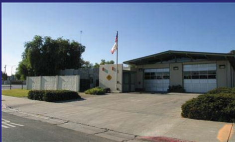
Fire Facilities Remediation
