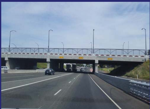
280/880/Stevens Creek Interchange Upgrade
