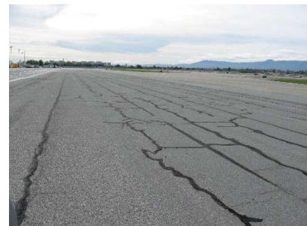
Southeast Ramp Reconstruction
