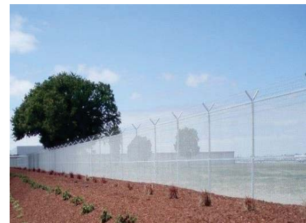
Perimeter Fence Line Upgrades
