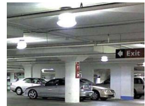
LED Garage Lighting Upgrades
