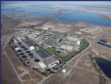
Water Pollution Control Plant
