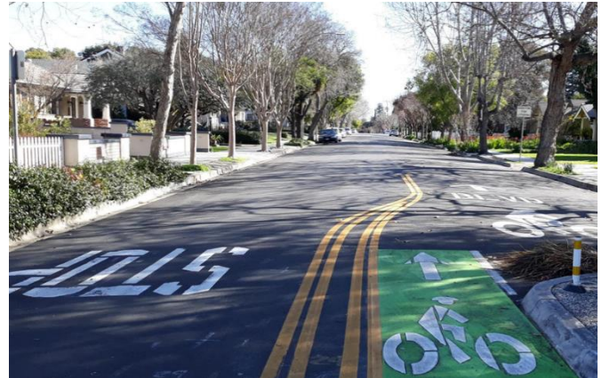
Sixteenth Street after resurfacing
