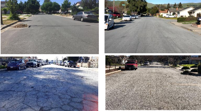
Clockwise from top left: San José streets in good, good-fair, poor, and failed condition
