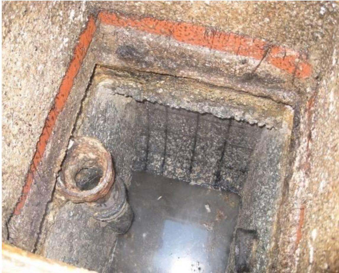
Rebar in Grease Interceptor
