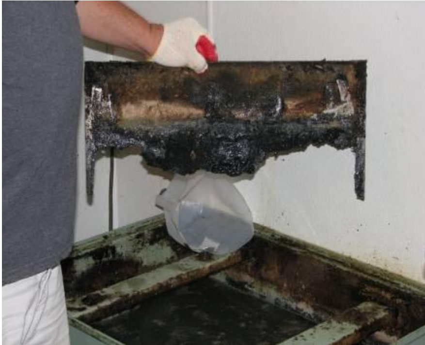
Corroded Baffle Plate
