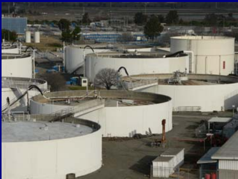
Digester Rehabilitation Project
