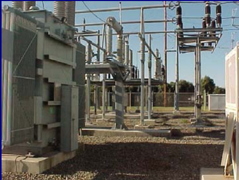
Plant Electrical Reliability Project
