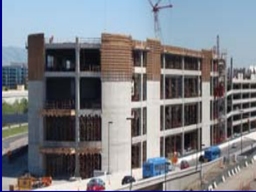
Consolidated Rental Car Garage
