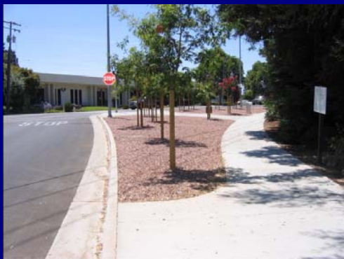
Hamilton Avenue Improvement Project
