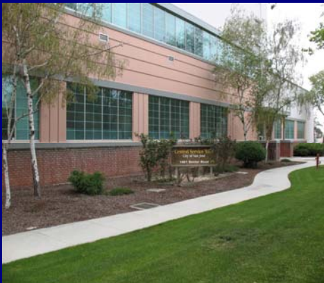
Central Service Yard
