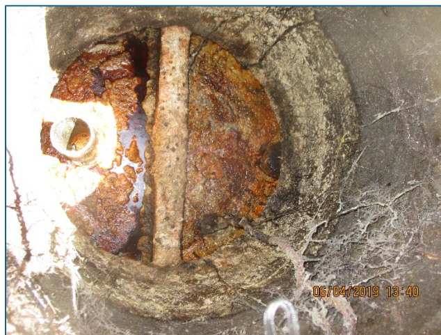
FIGURE 27. INSPECTING A COMMERCIAL GREASE INTERCEPTOR
