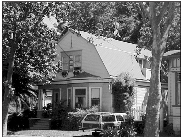
The Dutch Colonial Revival style in San Jose is easily identified by its Gambrel roof.
