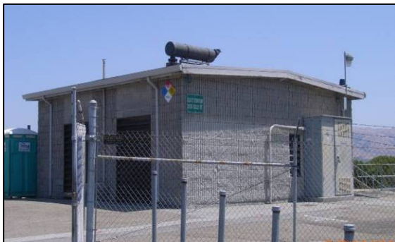
Gold Street Pump Station
