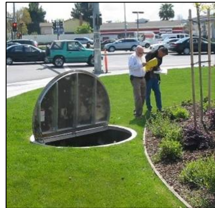
O & M Verification Program inspection of filtration vault
