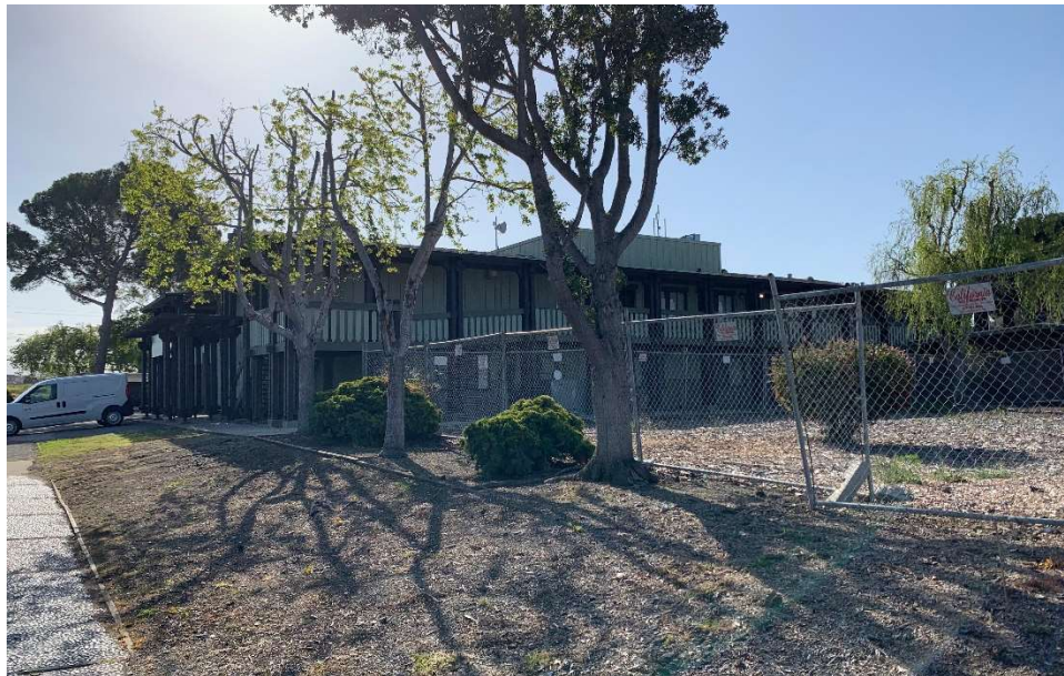
Figure 3. View of the building looking southeast from the corner of Hoppe and Gold streets. This image shows the fenced portion of the lot where the first Alviso Health Center building stood. It was removed between 2008 and 2011. Source: ESA, 2023
