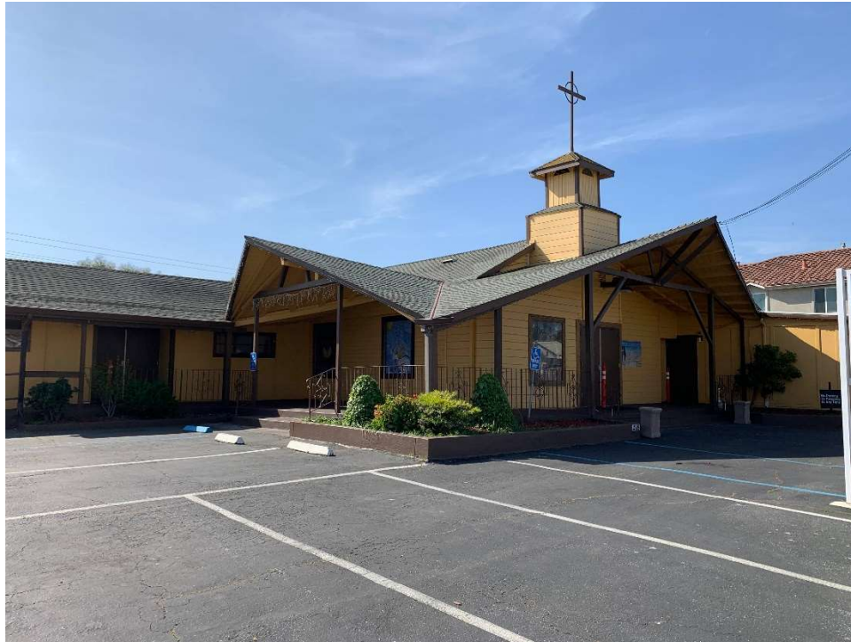
Figure 4. View of the butterfly porch roof. Source: ESA, 2023.
