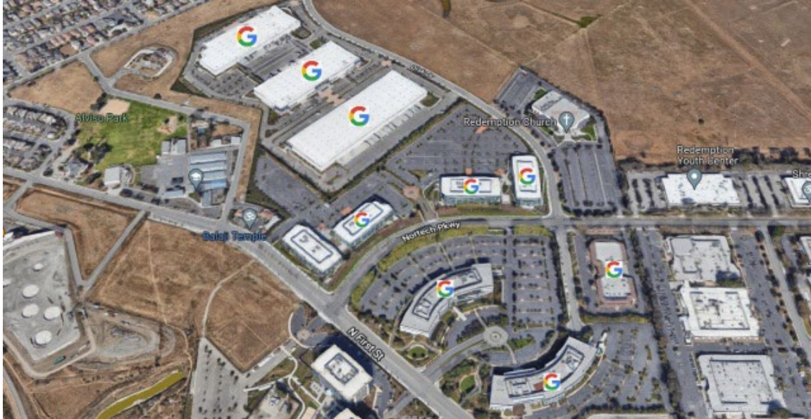
This aerial view faces north. The nine Google-owned buildings are identified with the multicolored “G” logos.
