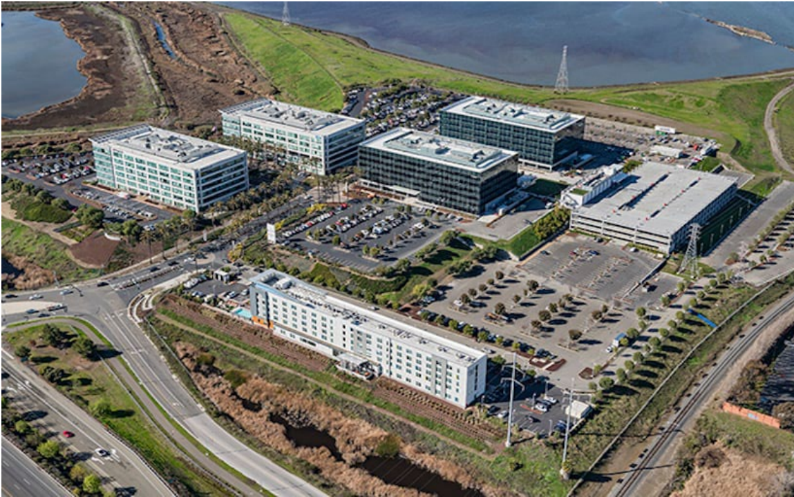
This aerial view faces northwest. Phase One included the two buildings on the far left, and Phase Two included the three buildings in the right background. Note that the Aloft Santa Clara Hotel in the foreground was not built as part of the America West campus.
