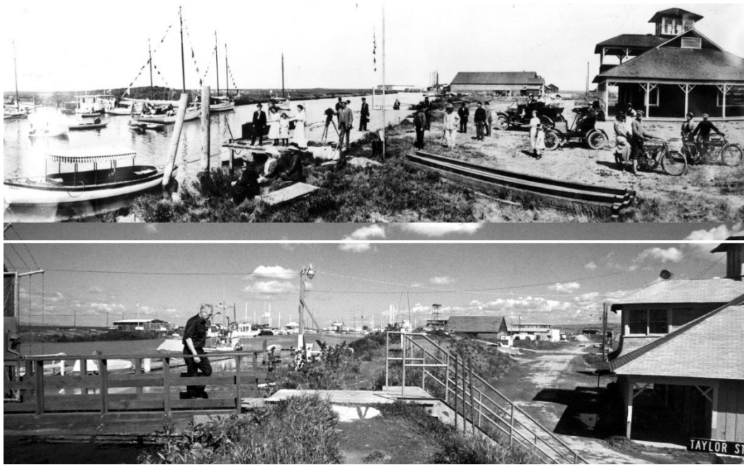
The upper photograph (taken ca. 1915) shows the South Bay Yacht Club at its original elevation and location at the corner of Hope and North Taylor streets. The lower photograph (taken in 1970) shows significant subsidence of the clubhouse.
