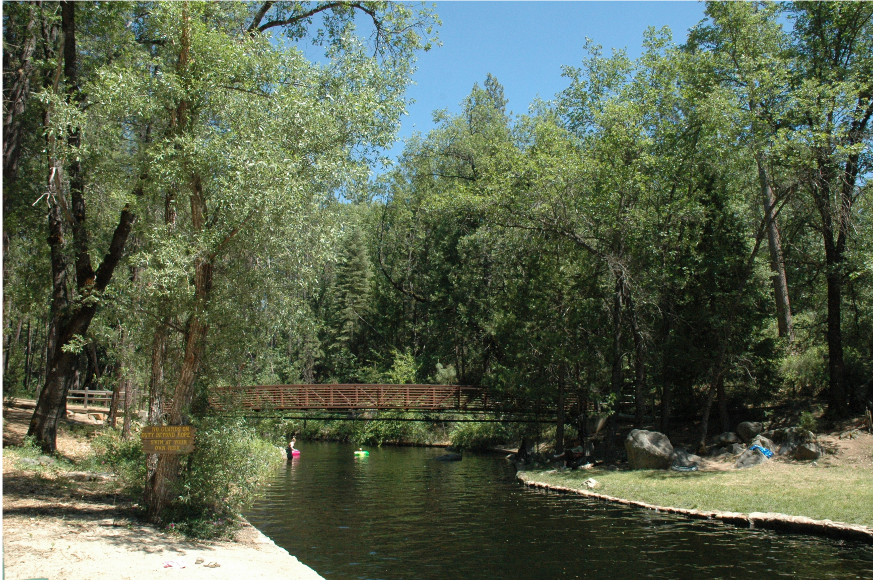
Upper Pedestrian Bridge Over the Middle Fork of the Tuolumne River
