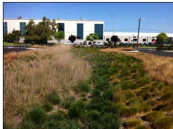
San José Environmental Innovation Center parking lot draining to a vegetated swale
