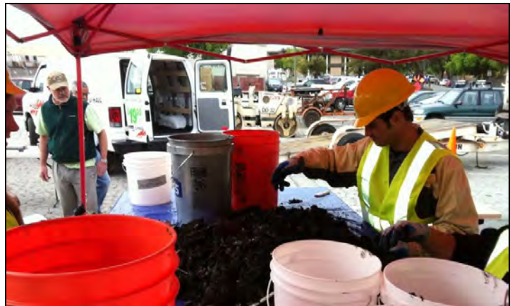
BASMAA contractor sorts through storm drain inlet debris at City of San José's Mabury Corporation Yard to quantify trash for baseline loading assessment
