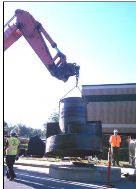
Hydrodynamic separator unit is placed into position on Wool Creek Drive
