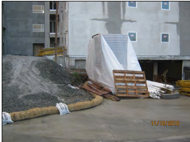
Good site management and sediment control at a construction site
