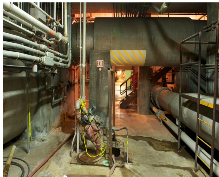
Figure 1: Existing service tunnels
