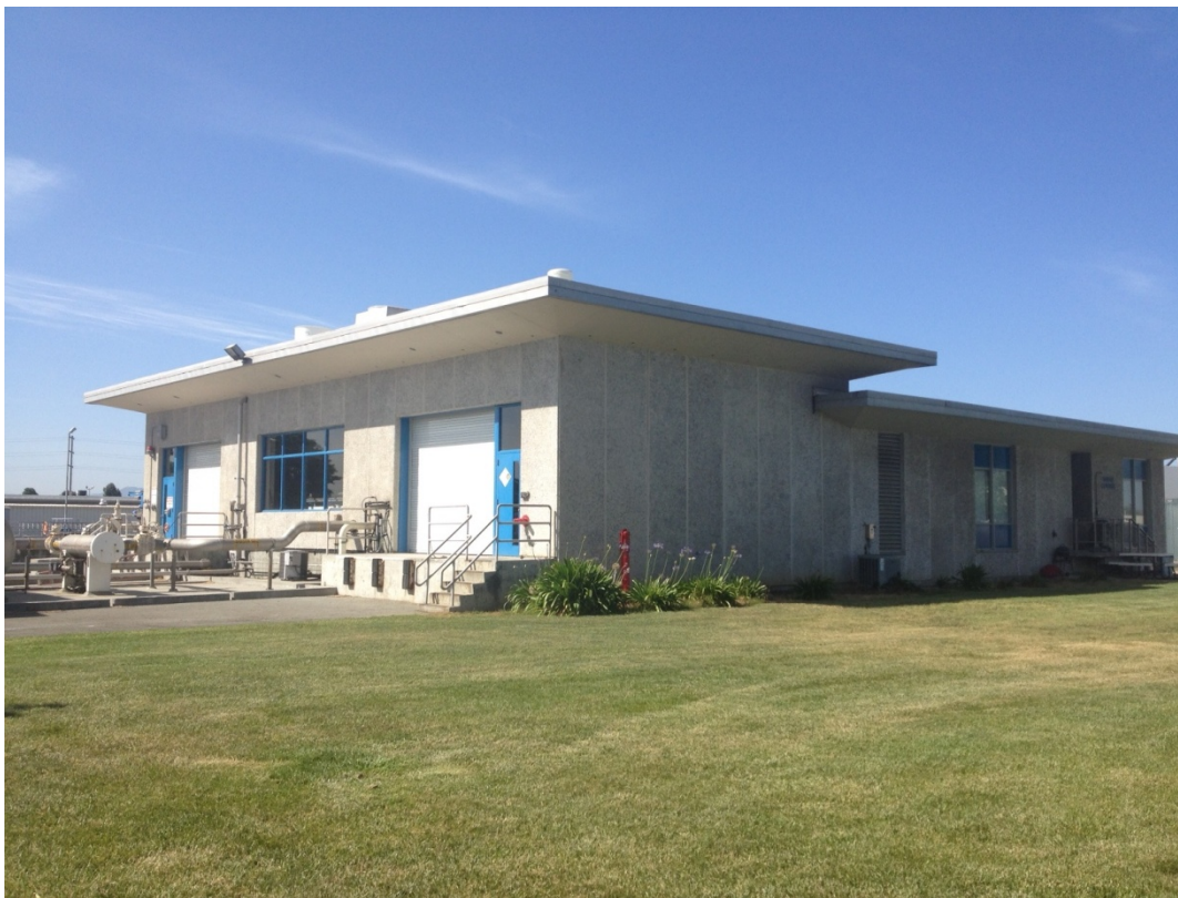
Figure 4: External View of Sludge Control Building
