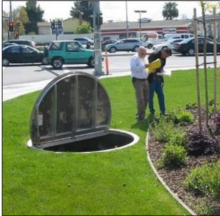
O & M Verification Program inspection of filtration vault
