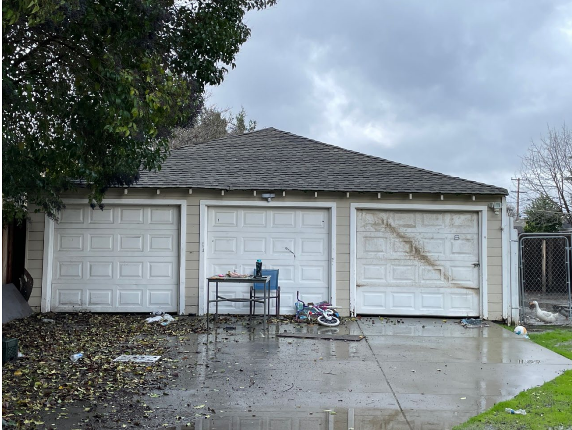
Photograph 4 1655 Lincoln Ave., San Jose View: front of 3-car garage constructed in 1952
