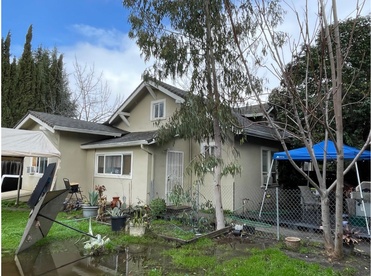
Photograph 3 1655 Lincoln Ave., San Jose View: Rear façade showing the multiple additions. Date: 1/12/2023
