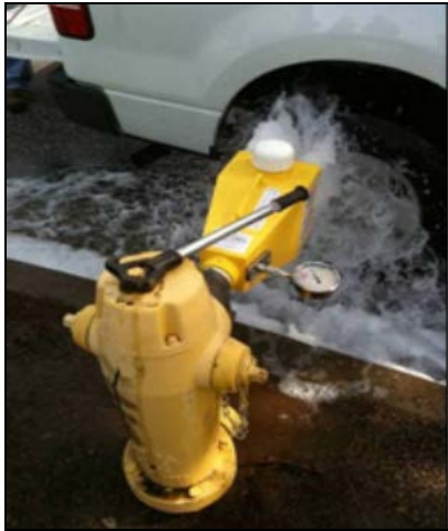
Potable water discharge BMP
