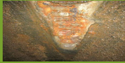
Existing condition of the pipe to be rehabilitated
