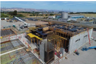
Overhead view of Dewatering Building
