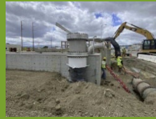
Milpitas Diversion Structure
