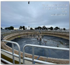
Contractor assembling the clarifier mechanism at nitrification clarifier B6
