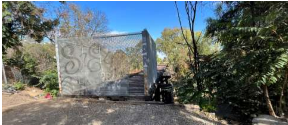
Figure 4. South entrance of Coyote Creek Trestle (September 2022).
