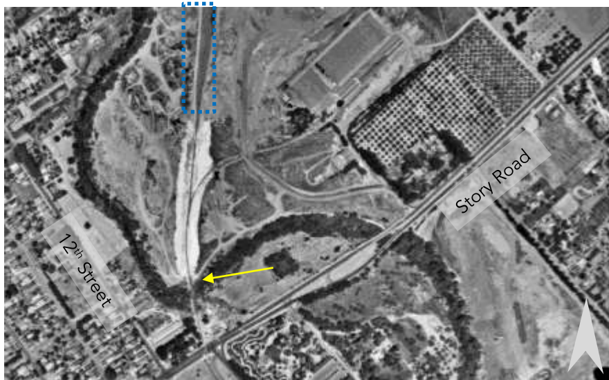
Figure 16. 1965 aerial photograph, the trestle pointed out with a yellow arrow, a partial view of the William Street Yard outlined in dashed blue (University of California, Santa Barbara Geospatial Collection).
