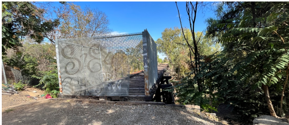
Figure 6. South entrance of Coyote Creek Trestle (September 2022).
