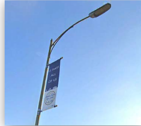
Streetlight Fixture Upgrade
