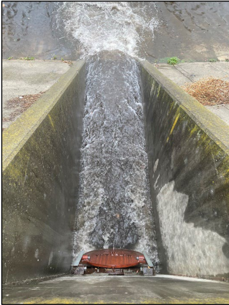
Wet weather PCBs/mercury sampling station at an outfall to San Thomas Aquino Creek
