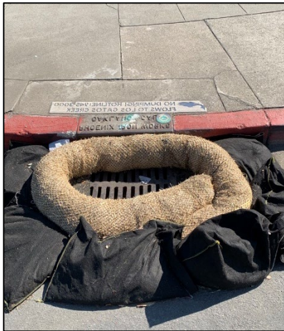
Effective BMPs installed at construction site.
