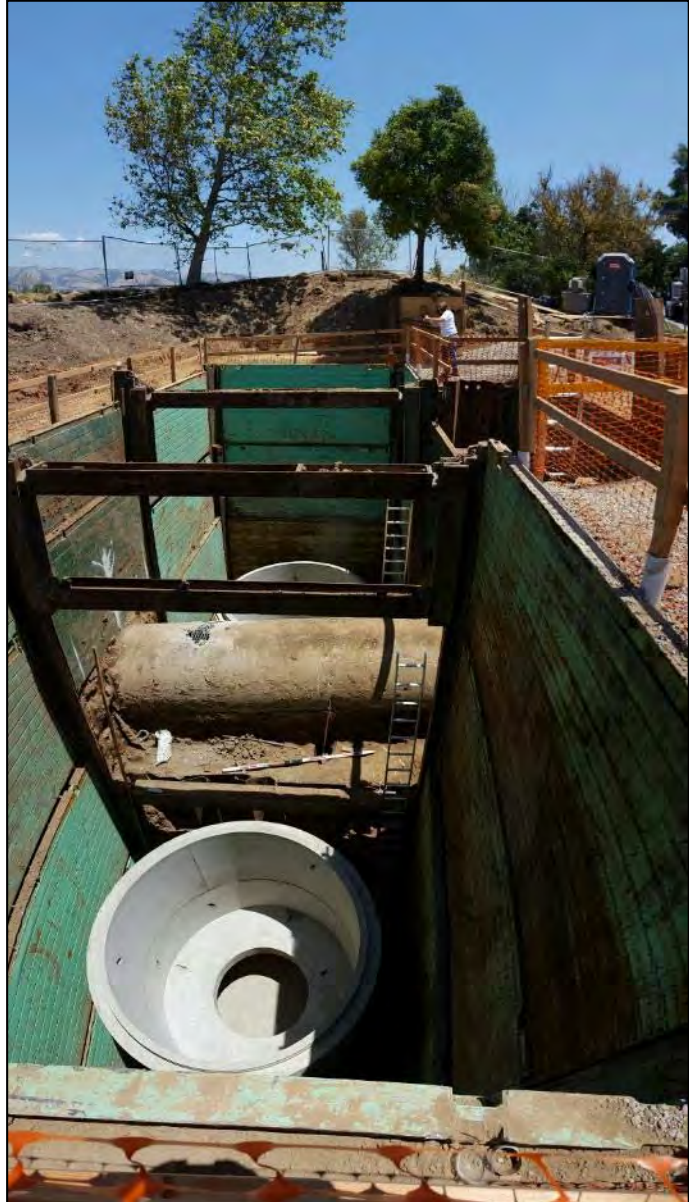
Twin CDS Unit Installation
