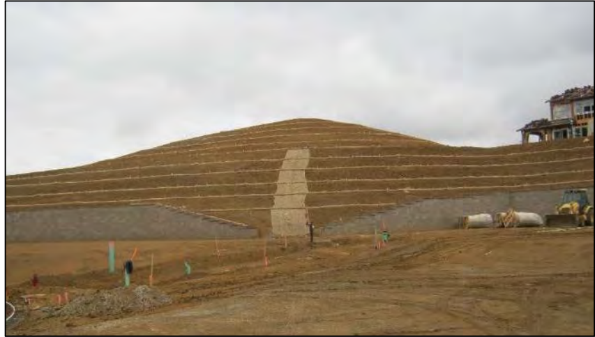
Steep hillside stabilized with wattle and ready for hydroseeding
