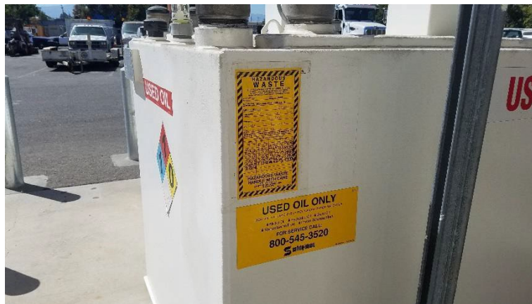
Figure 13: Hazardous waste identified with accumulation dates
