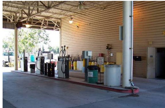
Figure 11: Example of BMPs: Absorbent and spill kits stored at fuel station
