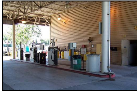
Figure 8: Example of BMPs: Absorbent and spill kits stored at fuel station
