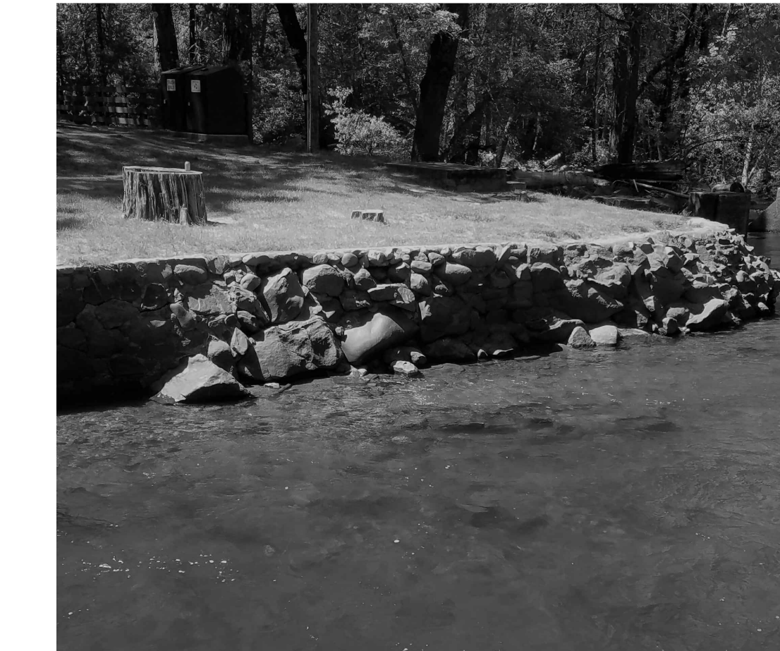
PHOTO #9: EXISTING SOUTH POOL STONE RETAINING WALL
