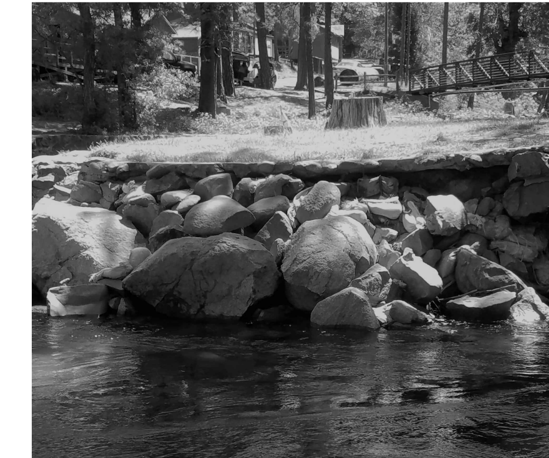
PHOTO #8: EXISTING SOUTH POOL STONE RETAINING WALL
