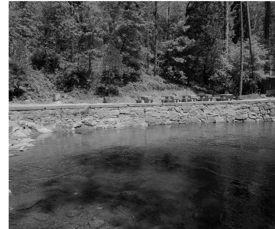
PHOTO #6: EXISTING NORTH POOL STONE RETAINING WALL
