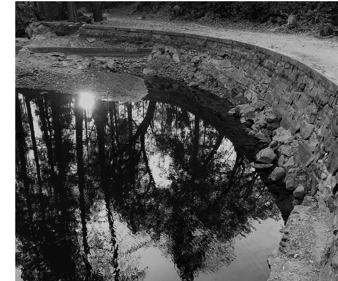
PHOTO #7: EXISTING NORTH POOL STONE RETAINING WALL
