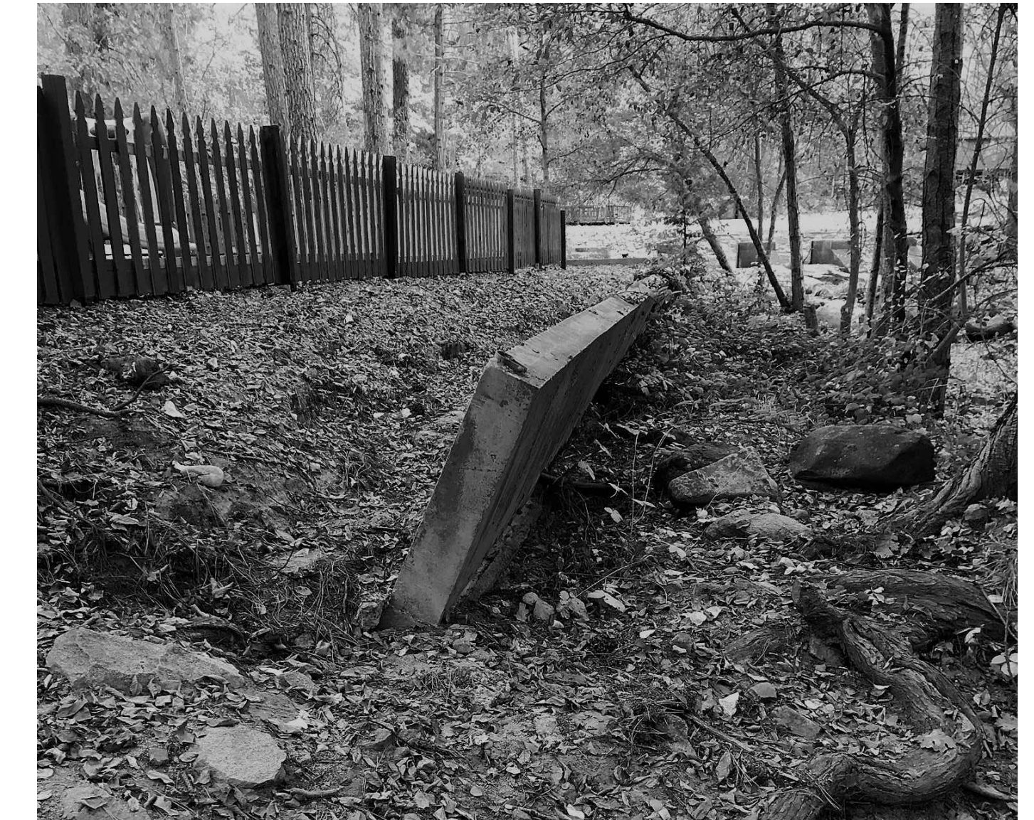
PHOTO #4: EXISTING CONCRETE RETAINING WALL
