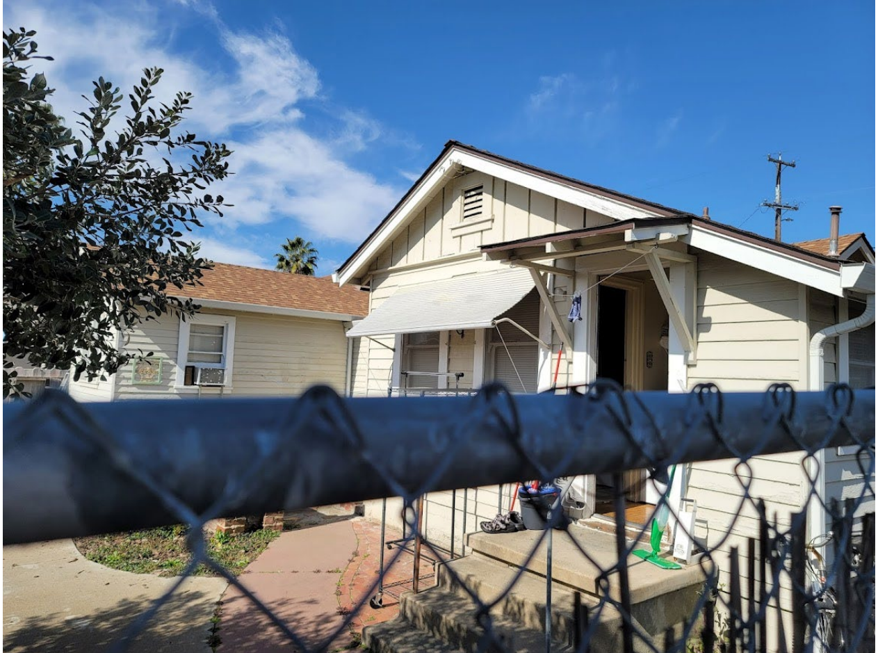
Photograph 4 125 Kirk Ave. San Jose View: Rear showing the two enlarged wings of the building. Date February 19, 2022
