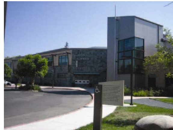
Almaden Multi-Service Hub Community Center Source: City of San José Greenprint 2009
