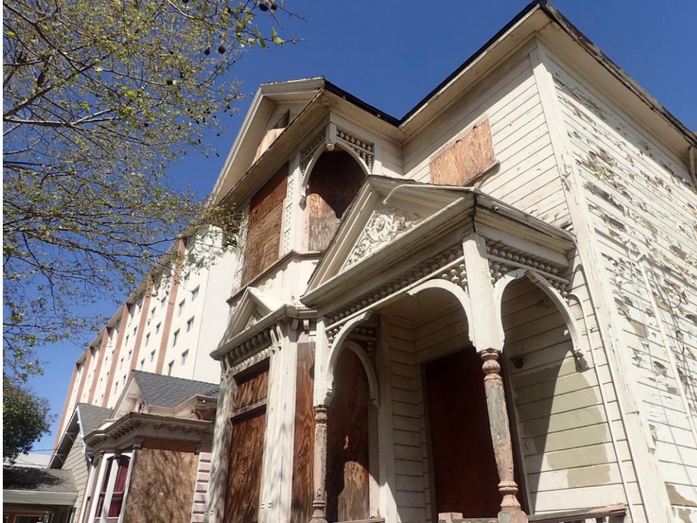
Detail view of front entry, viewed facing northeast.
