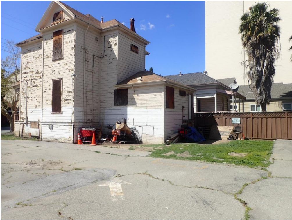
South side elevation, viewed facing northwest.
