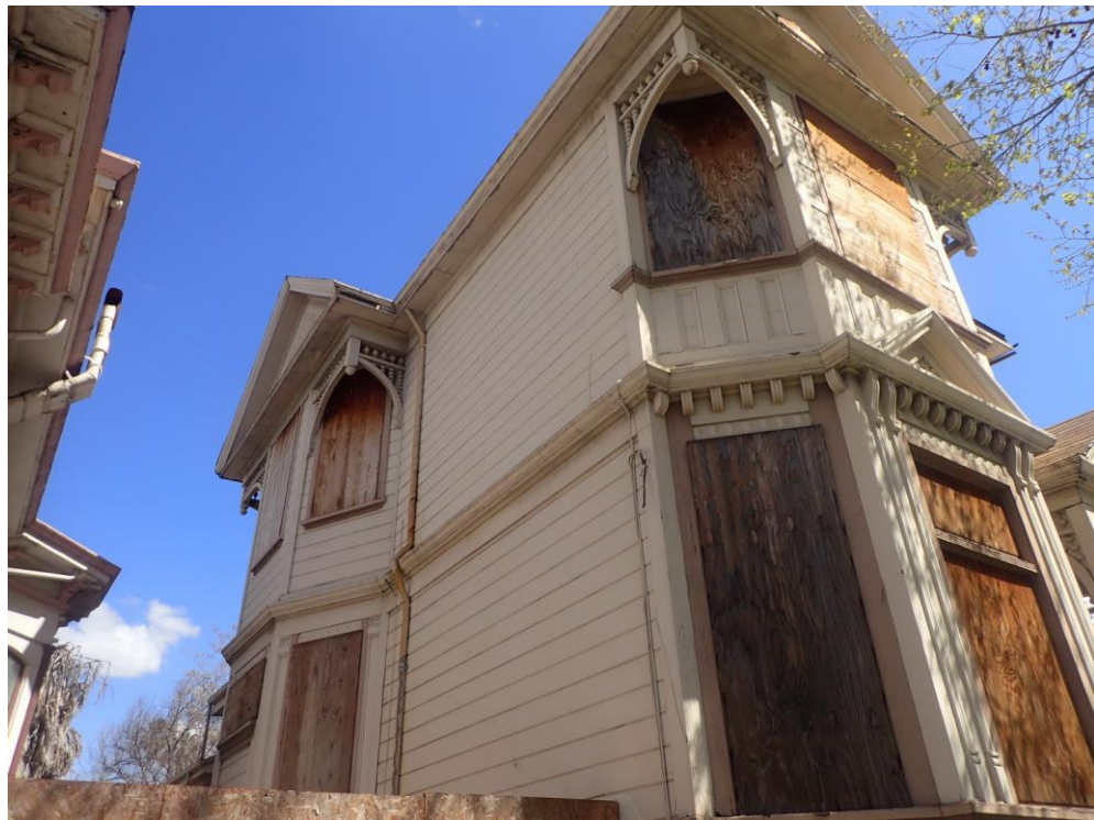
Detailed view of front and side bays, viewed facing southeast.
