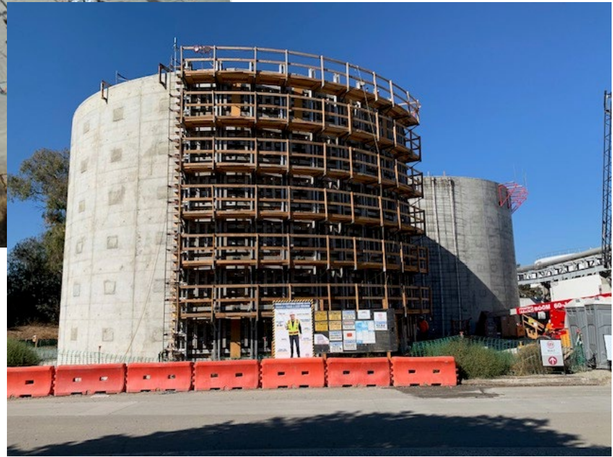
Sludge holding tank wall construction
