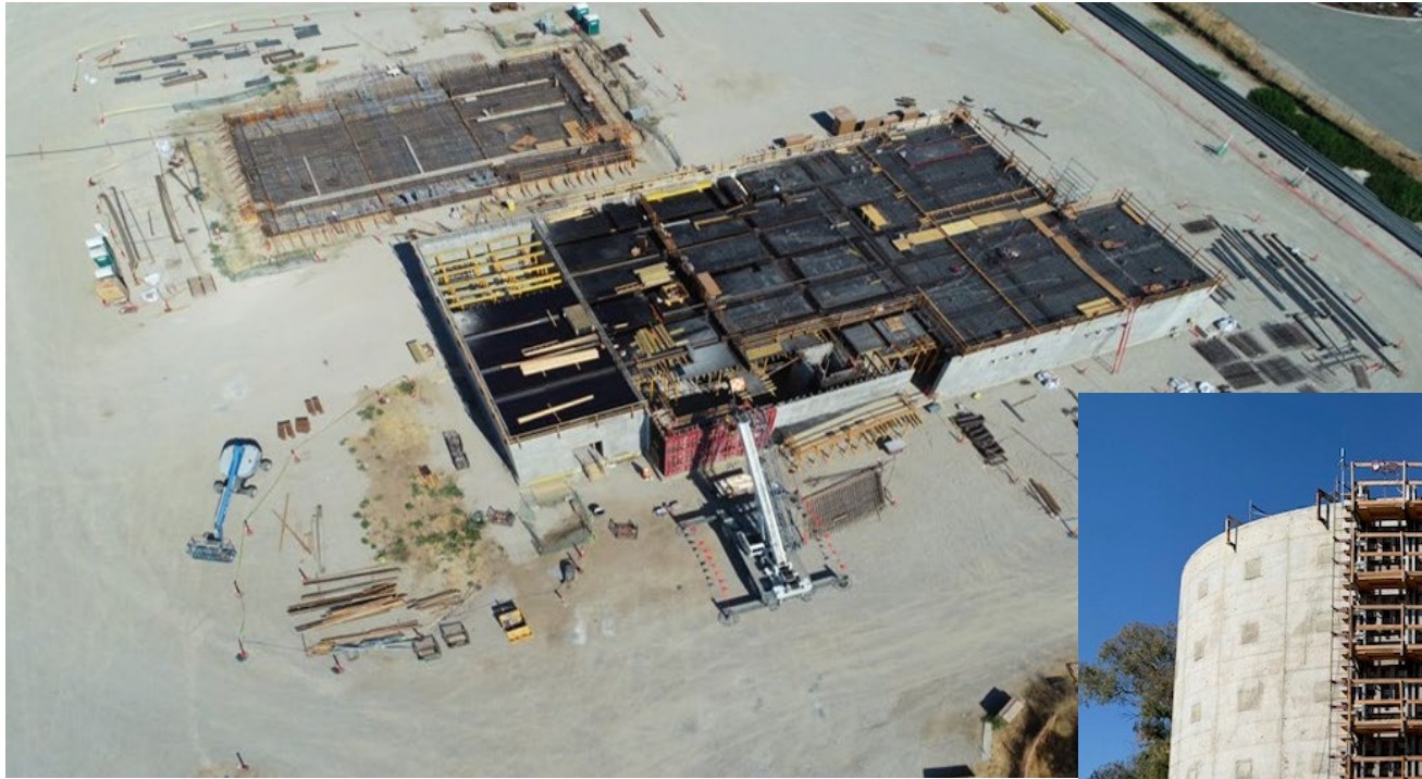
Dewatering Building completed walls Truck Load-Out slab-on-grade rebar installation
