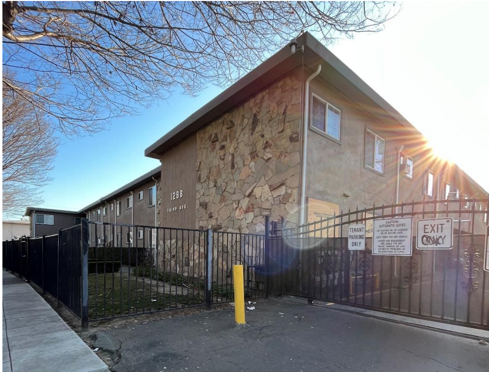
Figure 15. 1298 Tripp Avenue, view of the northwest and southwest façades (Image date February 2022).
