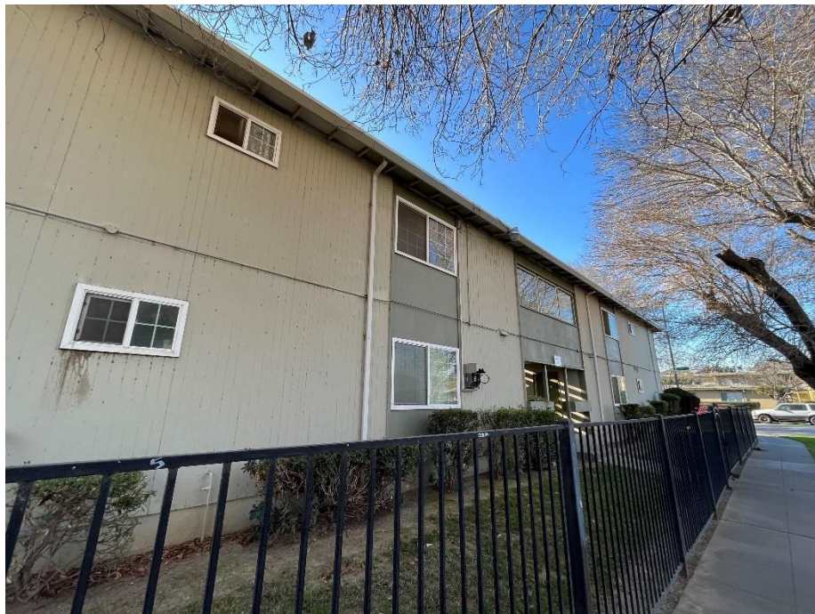
Figure 7. 380 N. 26 th St., northwest elevation (Image date February 2022).
