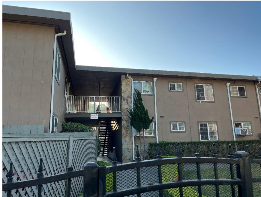
Figure 17. 1298 Tripp Avenue, northwest façade (Image date February 2022).
