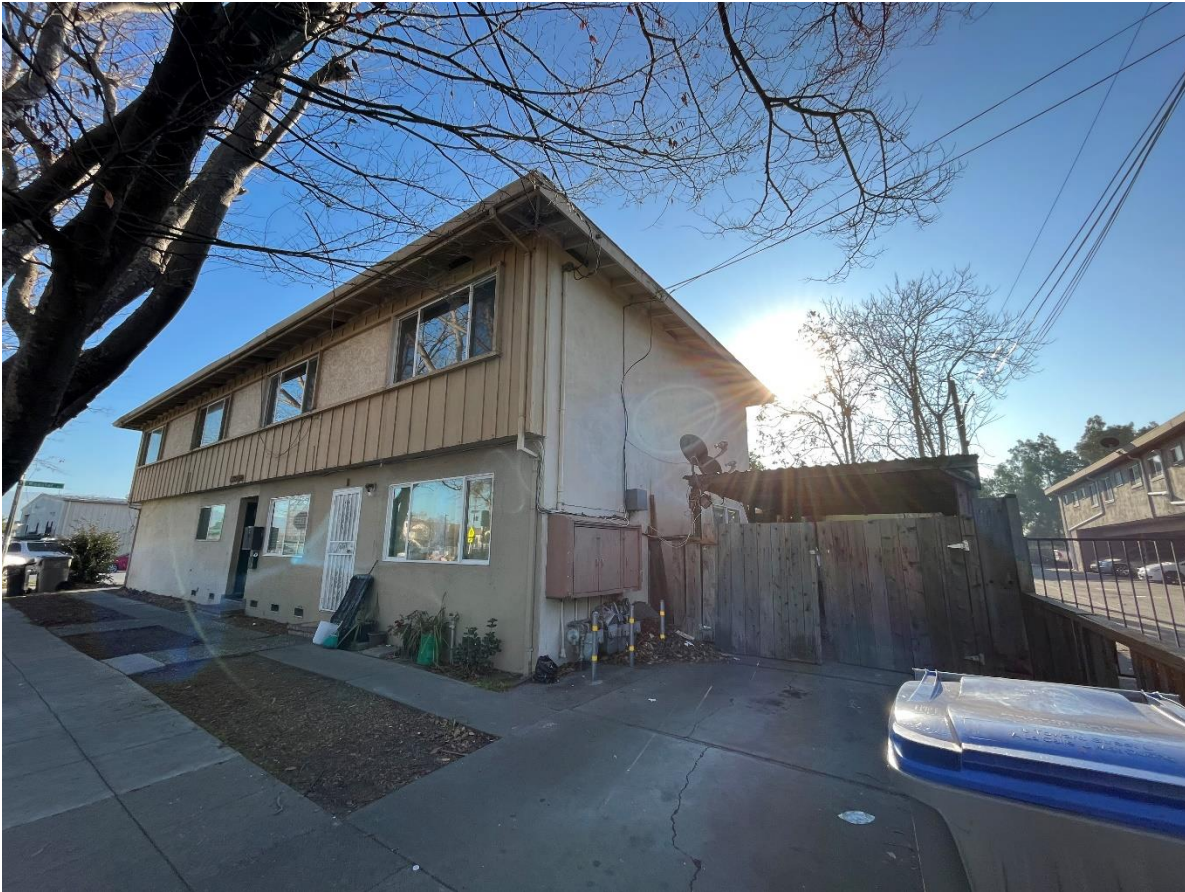
Figure 9. 1342 Tripp Avenue, northwest and southwest elevations with the shed (Imagery date February 2022).
