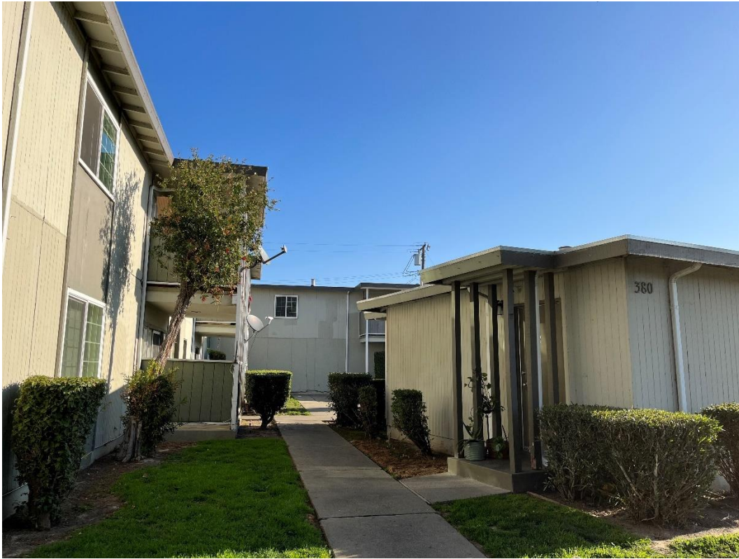
Figure 6. Street view of 380 N. 26 th St., southwest elevation (Image date February 2022).
