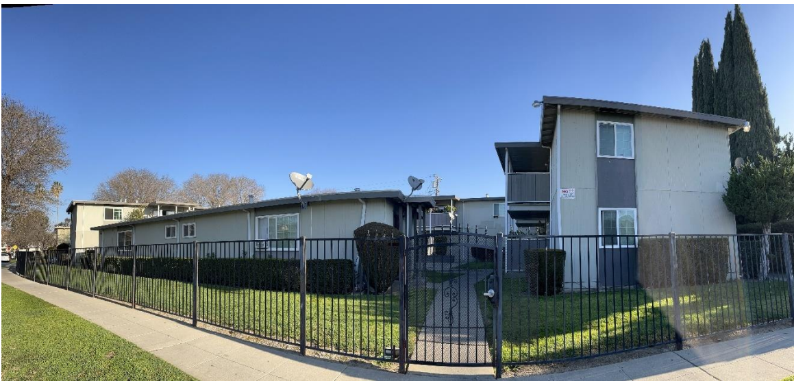
Figure 5. 380 N. 26 th St., southwest elevation (Image date February 2022).
