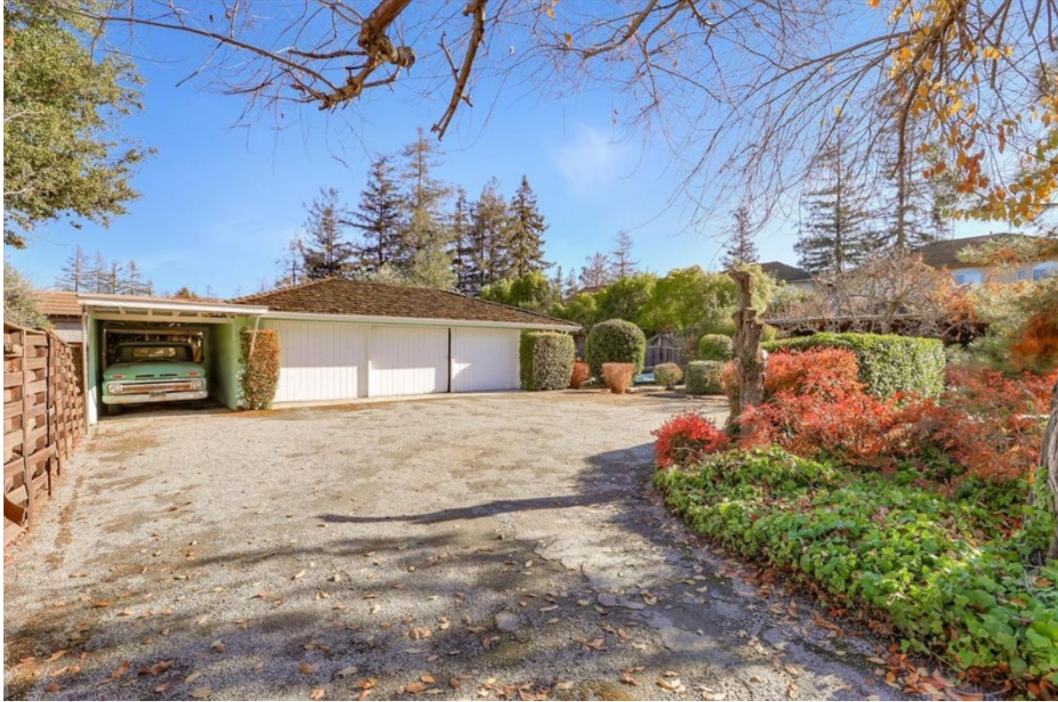
Photograph 4 1348 Miller Avenue, San Jose View: Three car garage and covered car port to the side and behind the main house.
