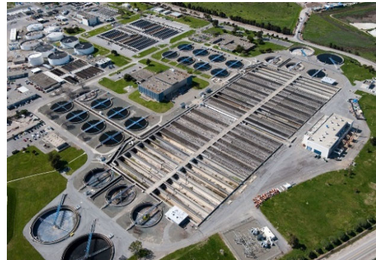
Aerial View of the San José-Santa Clara Regional Wastewater Facility
