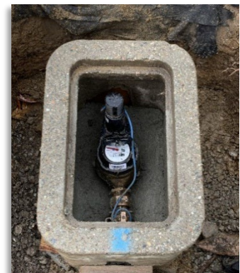
Installation of a new water meter box
