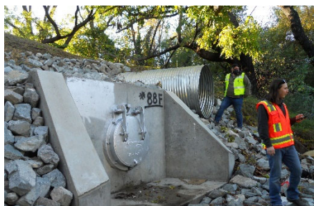
Storm Sewer Outfall
