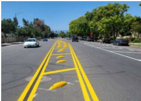
Illegal sideshow deterrents along Jackson Avenue including newly striped median and bike buffer
