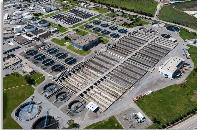
San José-Santa Clara Regional Wastewater Facility
