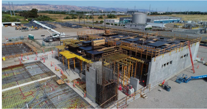
View of new dewatering building
