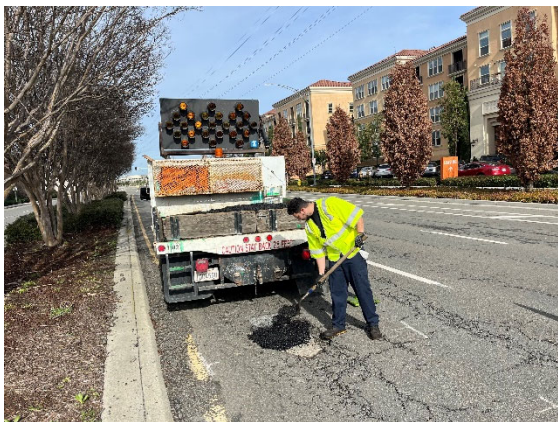
Pothole Repair
