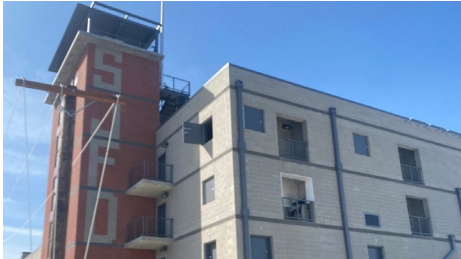
Completion of Fire Training Tower
