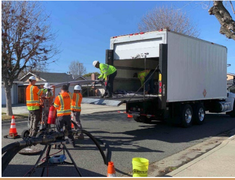
Sanitary Sewer Repairs Project (CIPP Liner Installation)
