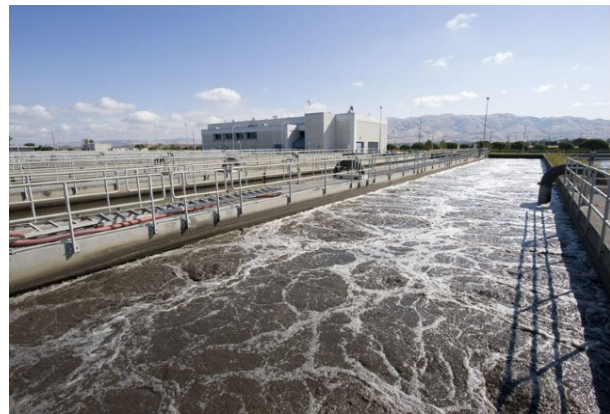
San José-Santa Clara Regional Wastewater Facility Aeration
