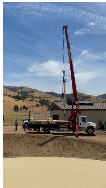
Installation of new pumps and motors at the Fowler Pump Station
