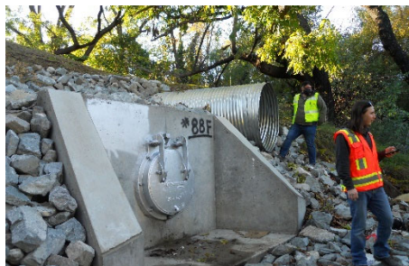
Storm Sewer Outfall
