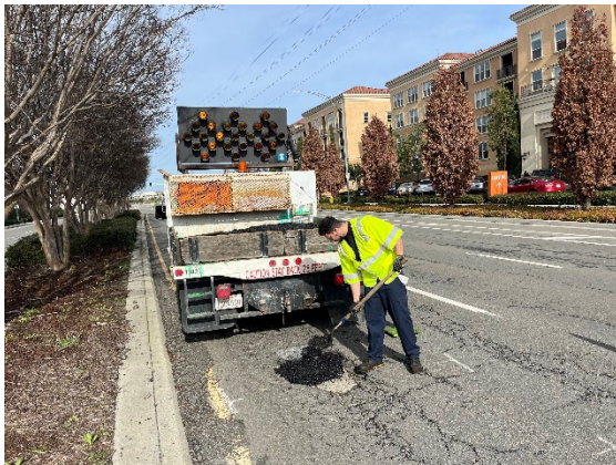
Pothole Repair
