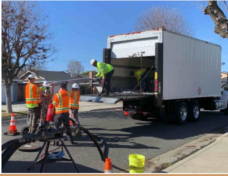
Sanitary Sewer Repairs Project (CIPP Liner Installation)
