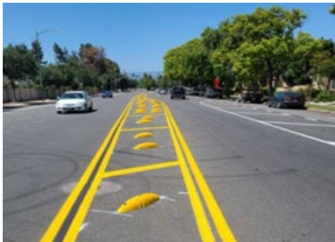
Illegal sideshow deterrents along Jackson Avenue including newly striped median and bike buffer
