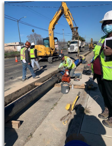
Construction of a main replacement project in North San José/Alviso
