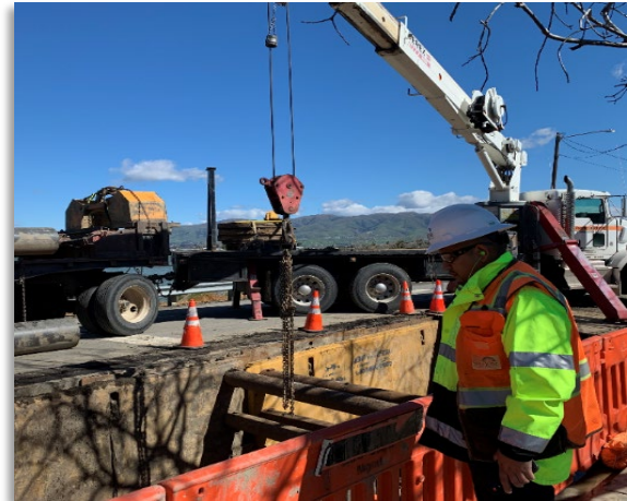
Preparing for a water main installation
