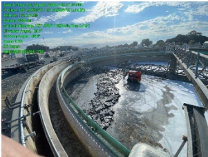
Grout removal within Clarifier B7
