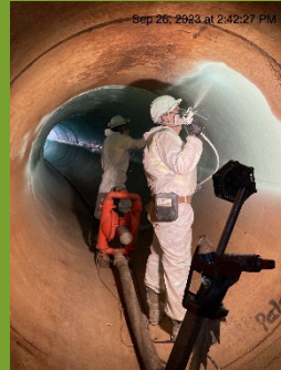
Workers applying an epoxy coating
