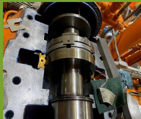
TBB Thrust Bearing Replacement – Thrust pad on right
