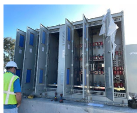
Assembly of S-6 Switchgear
