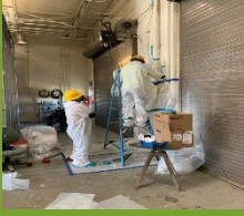
Paint shop lead mitigation
