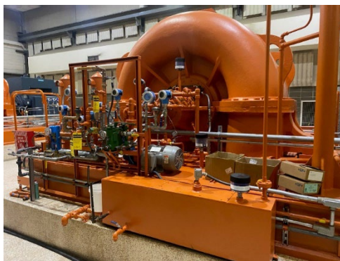
Tertiary Blower Building
