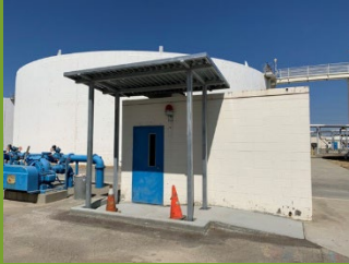
Tunnel canopy improvements
