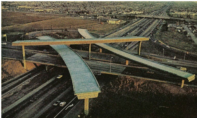
Figure 10: The 680, 280, and 101 freeway interchange, under construction in 1976
