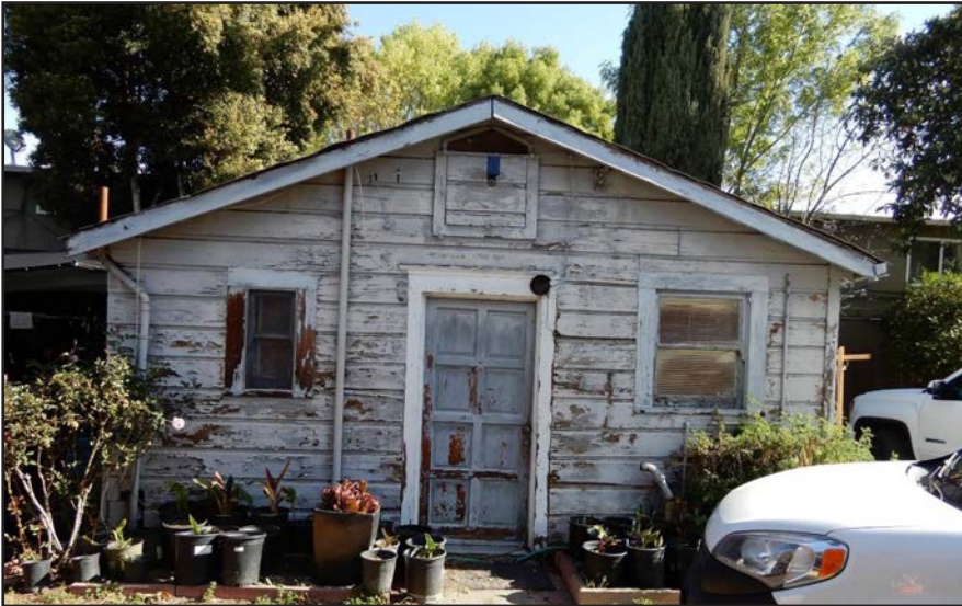
Photo #7: East facing view of accessory structure at 1279 East Julian Street.
