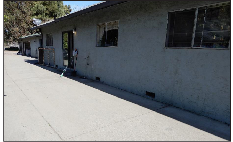
Photo #2: East facing view of 1271 East Julian Street from existing driveway.
