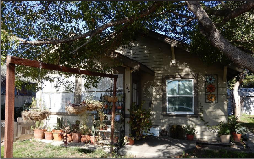
Photo #5: Northwest facing view of 1279 East Julian Street from front yard.
