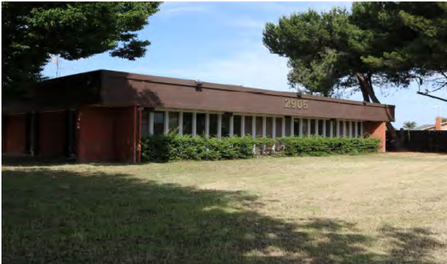
Photo 3. View of the existing KLOK radio station building at the northeast corner of the site.
