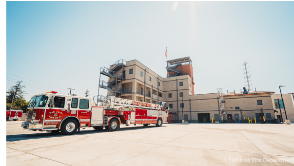
Source: San José Fire Department, photo of Fire Training Center
